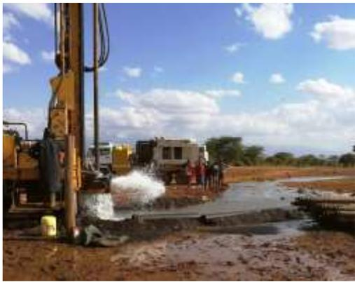
The Namelok community borehole was born on July 5, 2019 at 12:20 pm. We were blessed with our most productive well to date – the capacity is more than 50,000 liters / per hour. Water quality analysis confirmed that the water is perfect for human consumption - no salt, no fluoride or other chemicals.
